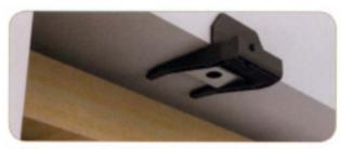
Take the tool and bracket to the window recess. Butt the flat vertical face of the tool against the outer face, and hold the bracket against the top face of the recess approximately 100mm in from either side of the recess.
