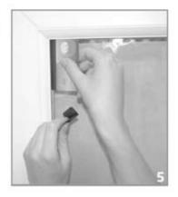
Line up the window fixing bracket at the base of the card (or top of the card depending upon which corner of the window you are working) and fit the bracket by pushing it between the glass and the rubber seal on the window.
