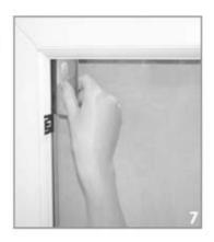
(3) Fit any intermediate brackets accordingly. Clean excess lubricant from window surface prior to fixing frame to brackets.
