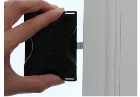
14. Position relevant number of recommended side extrusion clips according to the drop of the blind. Push home the extrusion clips with fitting tool.
