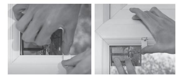
Once all brackets are in place the shutter is ready to be installed. Line the cutout in the bottom of the frame with the bottom brackets.
